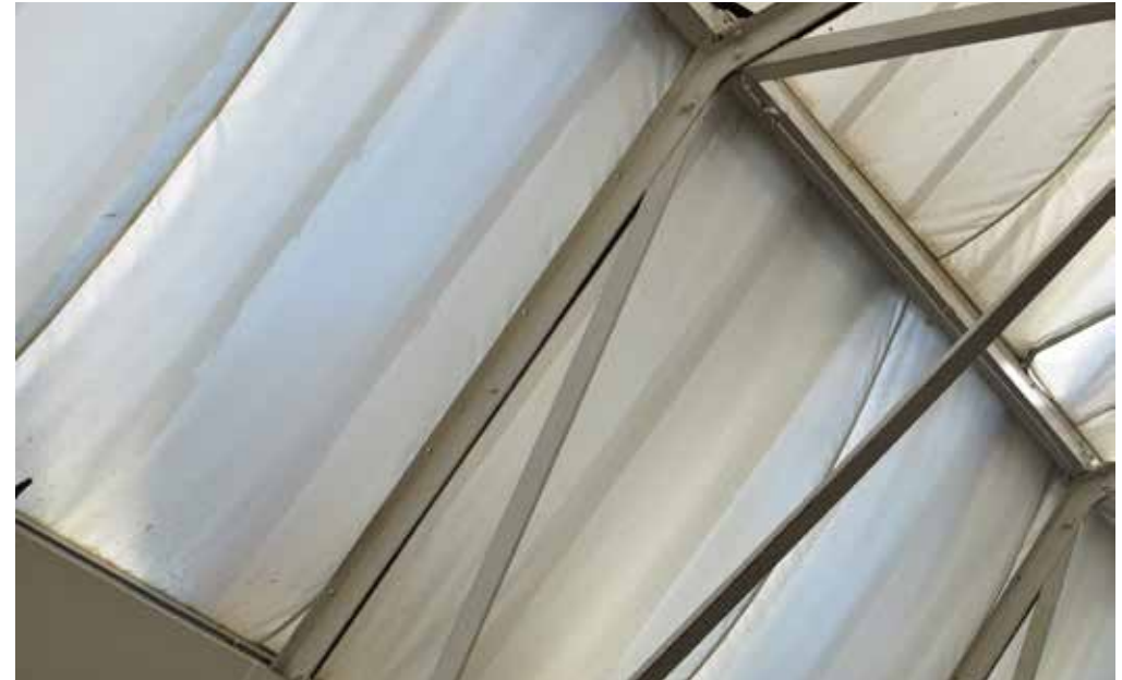
14. Redundant holes in steel for timber purlins showing area of glazing was increased.
