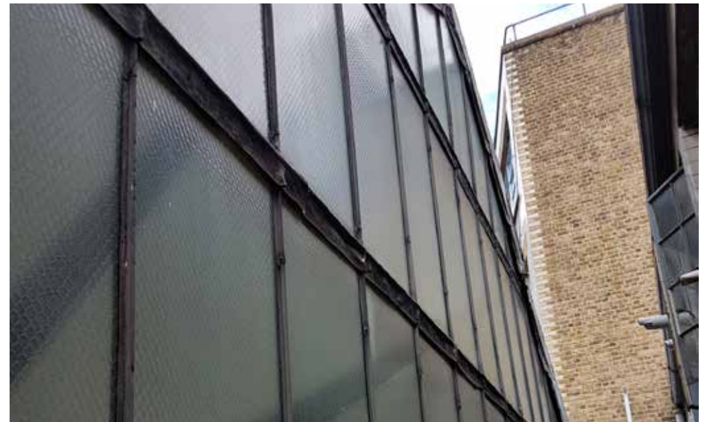
21. Patent glazing system to roof and early curtain wall glazing to gable with massive iron girder
