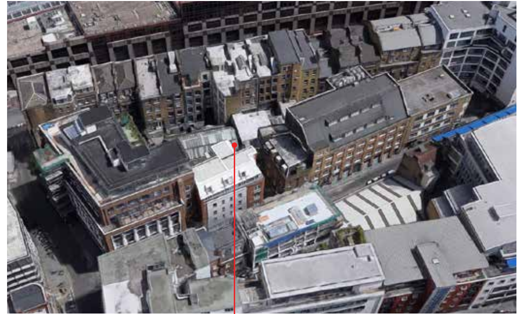
06. Birds eye view looking west | The Drill Hall
