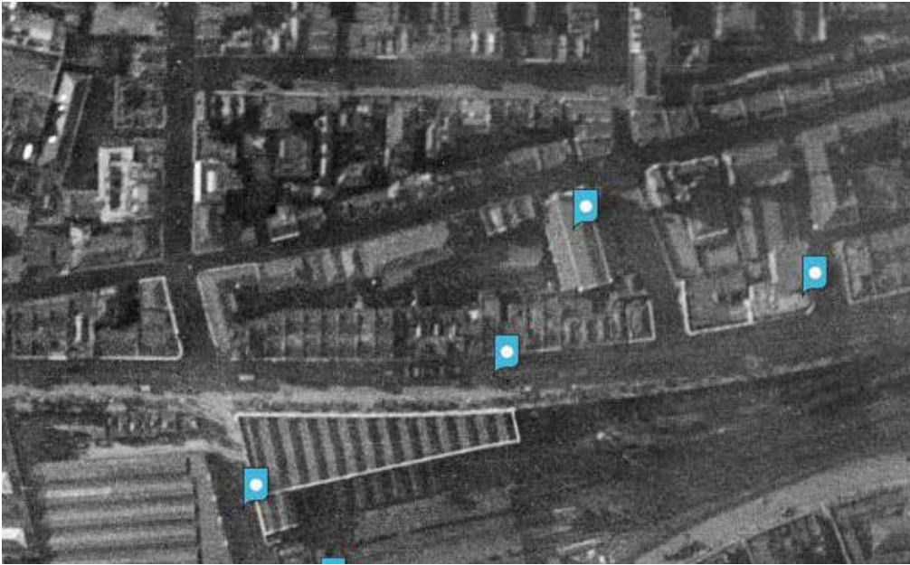
16. Aerial view 1920 appears to show 1 Lily Place without its extension
