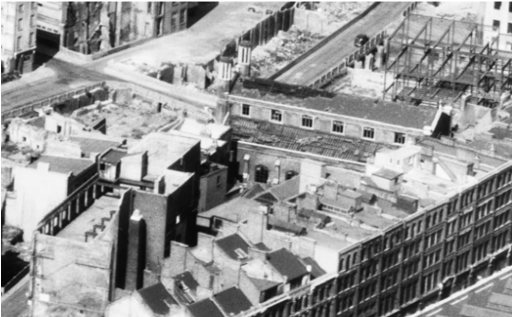
18. Bird's eye view 1947, showing extension to 1 Lily Place and gable wall to the Drill Hall
