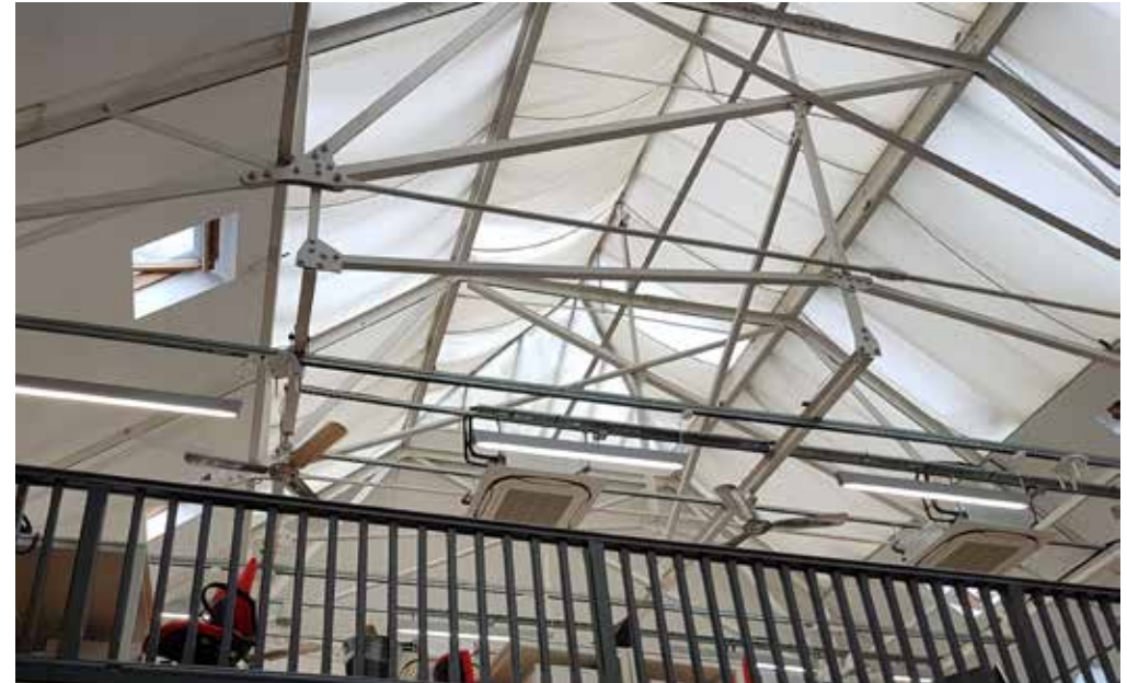
20. Original lightweight steel truss roof structure
