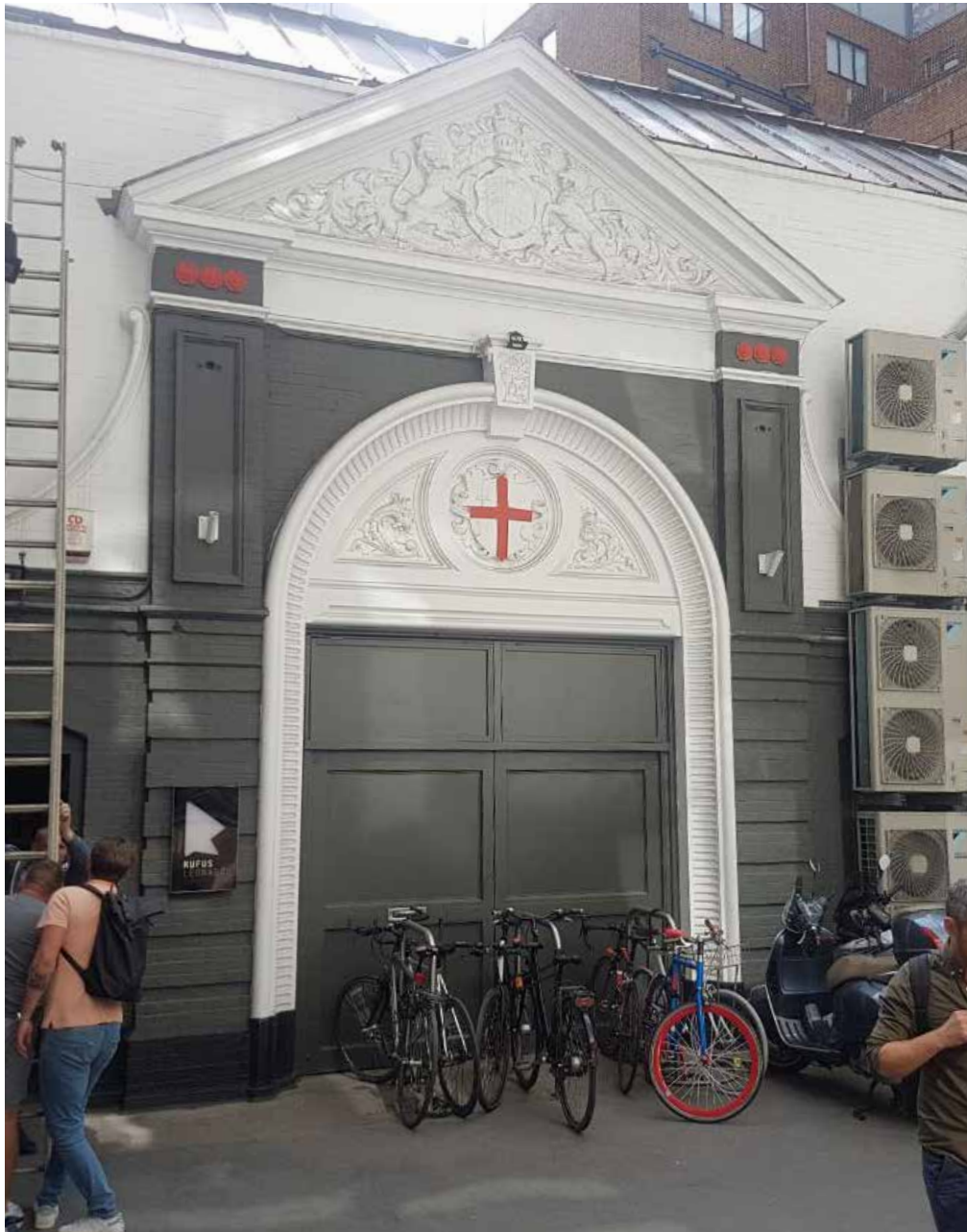
09. East elevation, accessed from Farringdon Road
