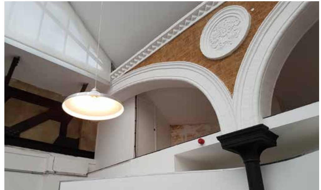
15. The original brick arches bisected by the glazed gable and wrought iron girder to 1 Lily Place
